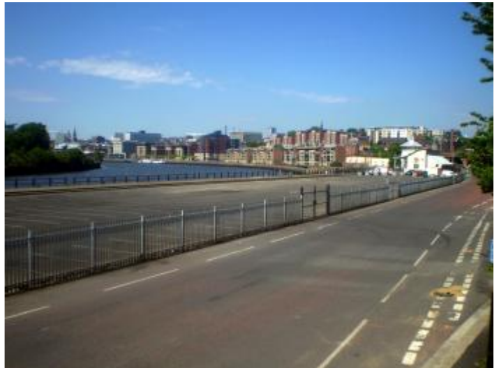
Spiller's Quay and Boathouse
